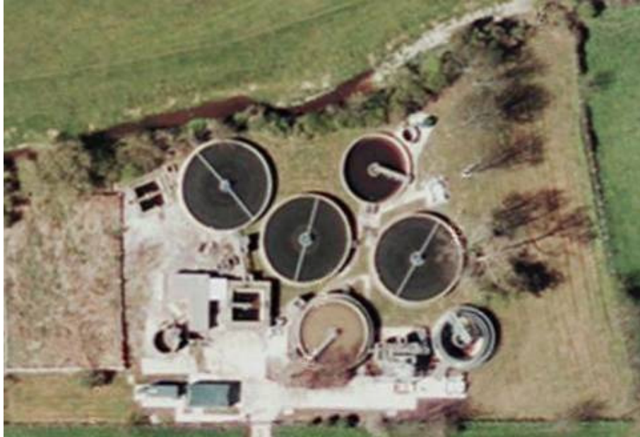
Figure 9 – Aerial Photo of Lavant WwTW
