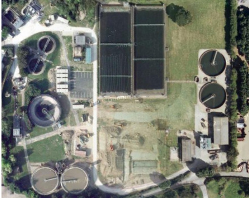
Figure 8 – Aerial Photo of Thornham WwTW
