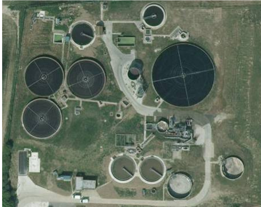
Figure 5 – Aerial Photo of Pagham WwTW
