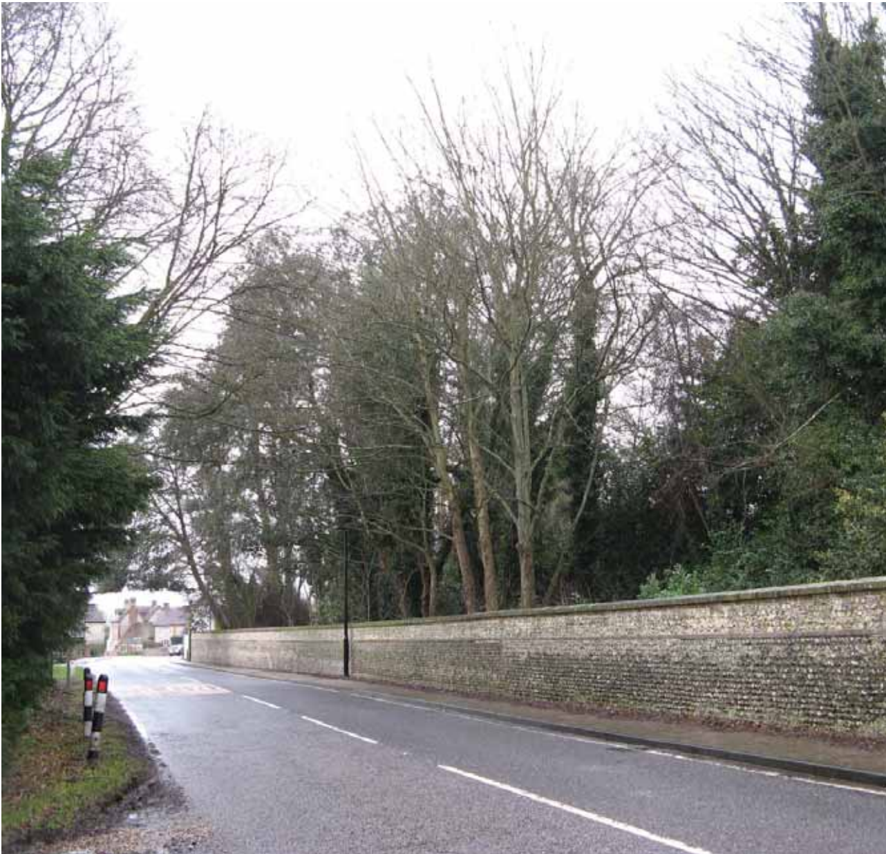
Flint boundary wall to Halnaker House
