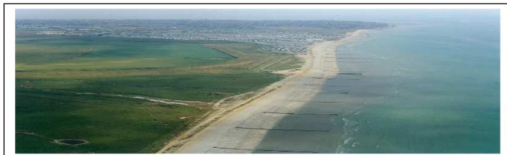
Figure 3.1 The Manhood Peninsula coastline looking along the Medmerry frontage towards Selsey
