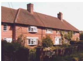
Greengates, 1st Tranche.
