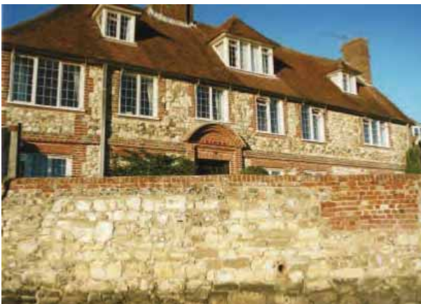
The Old Town Hall (Chandlers House)
