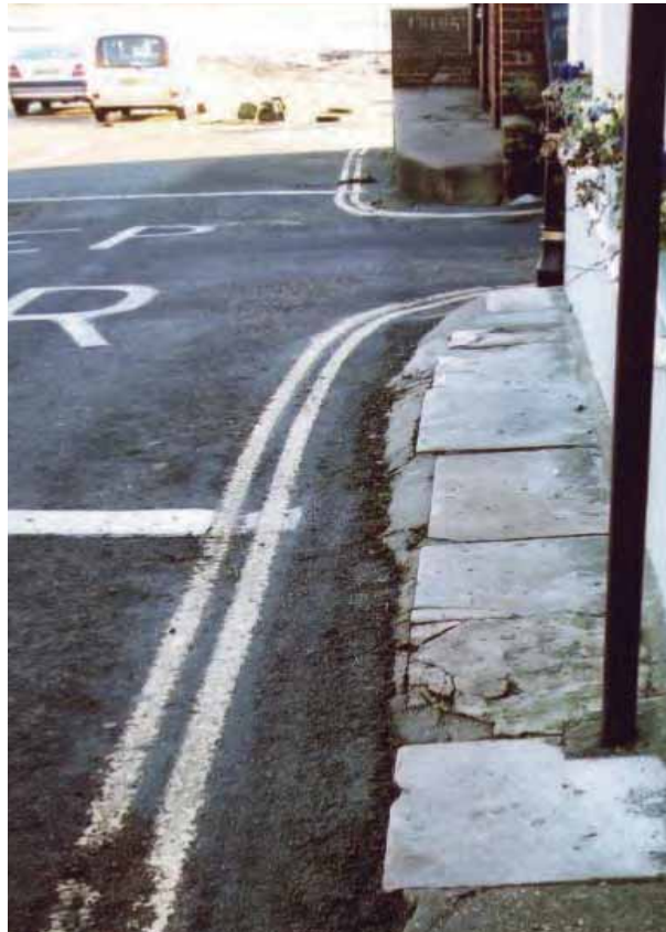
Pennant stone paving in Bosham Lane
