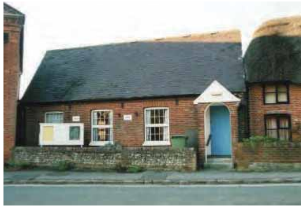
Slate roofs (former school, Bosham Lane)
