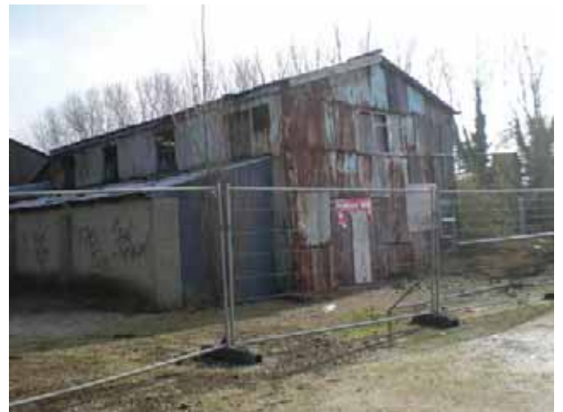
Derelict land to north of Bosham Conservation Area
