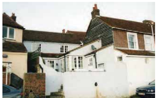
Back elevations to listed High Street properties
