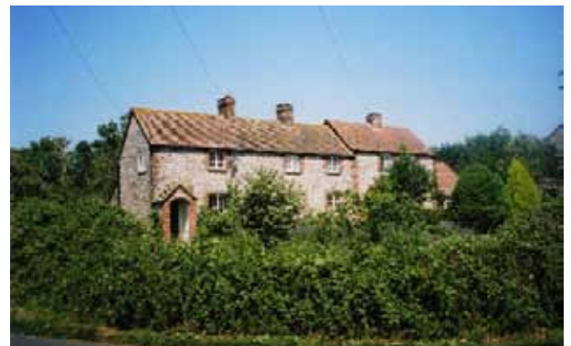
Nos. 1, 2 and 3 Church Cottages
