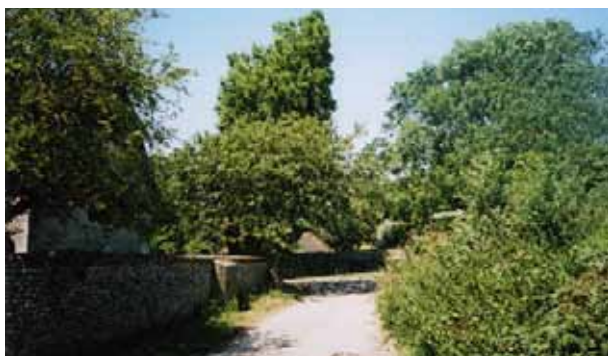
The road around the church is in poor condition
