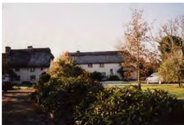
Cottage Row, Hundredsteddle Lane (on left)
