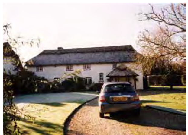
The Old Court House, Hundredsteddle Lane
