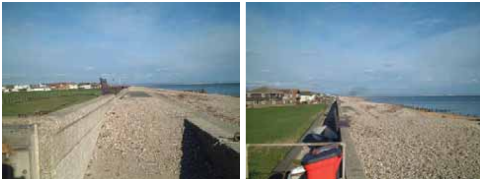
Photos: Difficult Access & Movement – Seawall, Selsey
