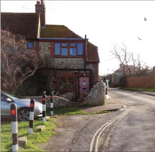
Flood wall on Albion Road East
