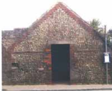
The stone bus shelter
