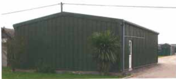
A modern metal shed whose visual impact will be improved when the trees and bushes have grown
