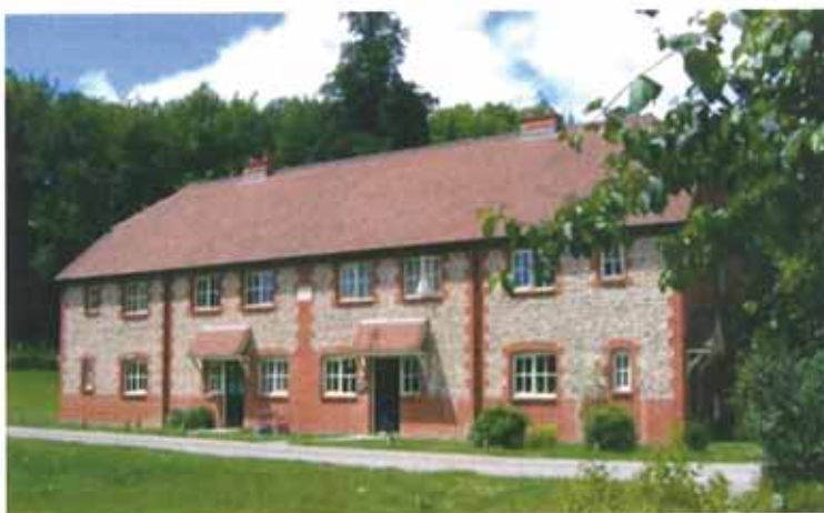
Affordable housing at West Dean College, West Sussex in a design suitable for Sidlesham.
