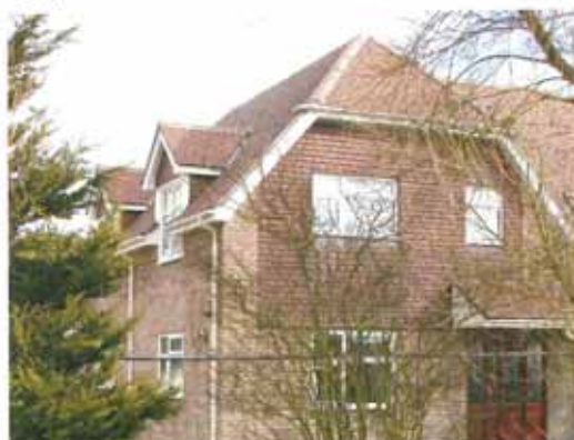
Dormers and a Sussex Hip (but inappropriate eaves)
