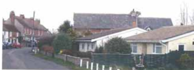
Bungalows which do not fit ideally in Mill Lane
