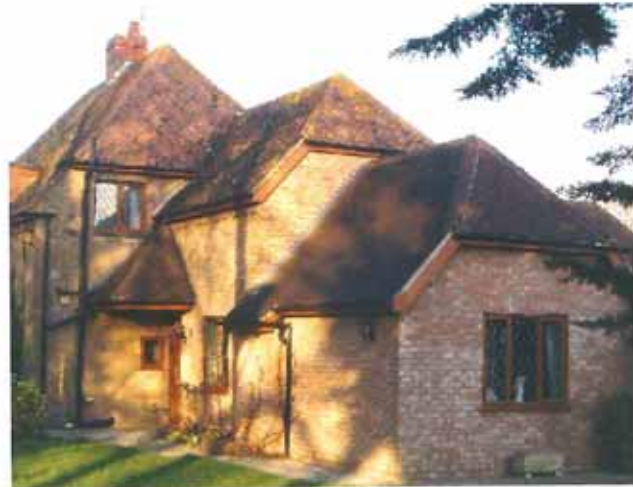
A good example of extensions and suitable windows
