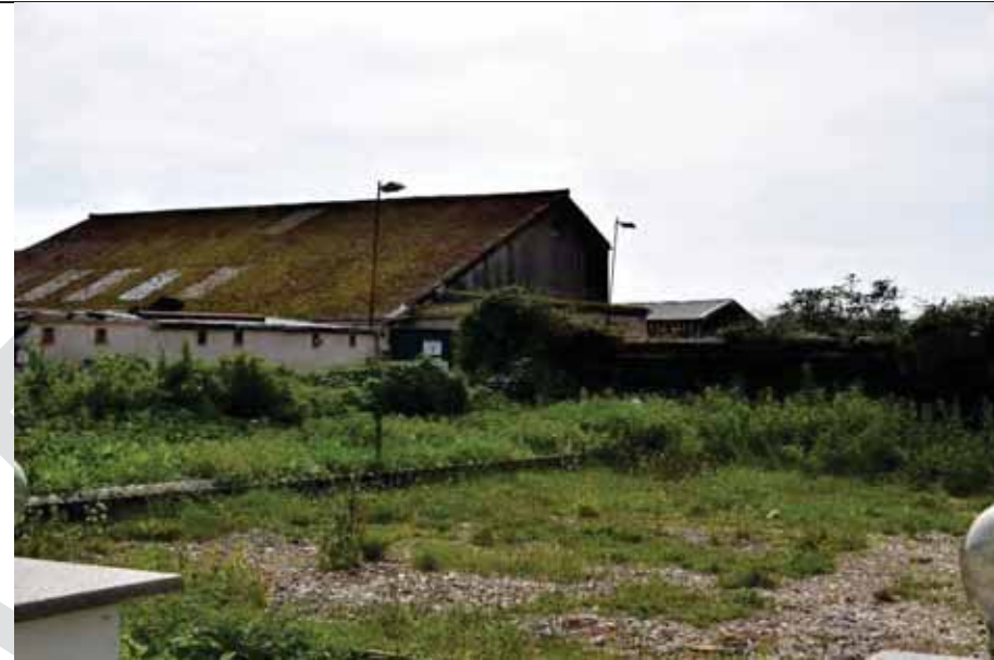
Photo 3: View south-west from adjacent to India Gate, Green Lane into Kives Farm
