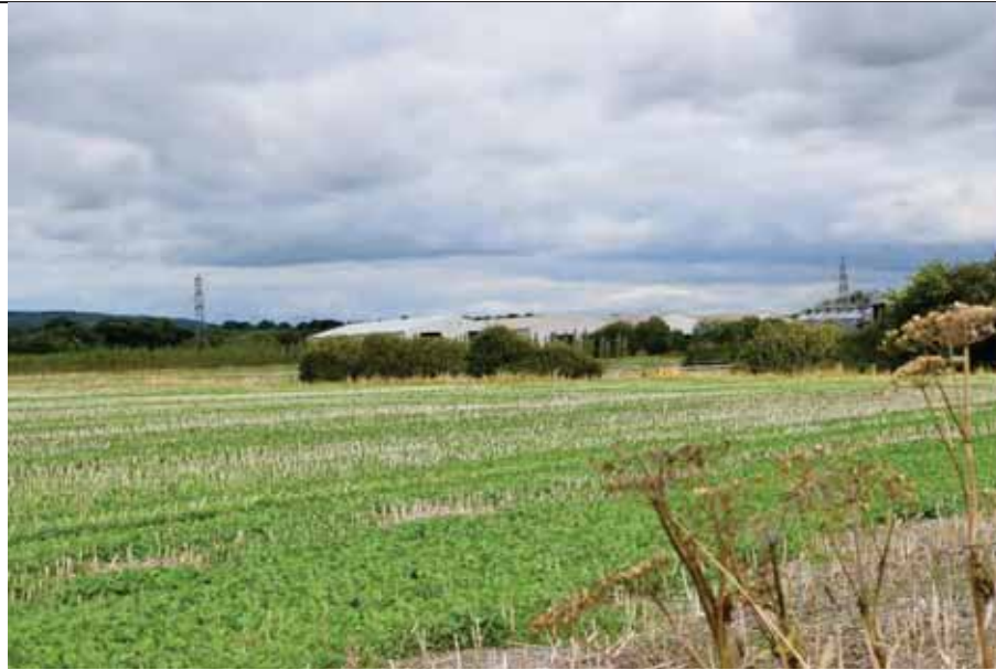
Photo 4: View from Priors Leaze Lane looking north to large farm buildings at Priors Leaze Farm
