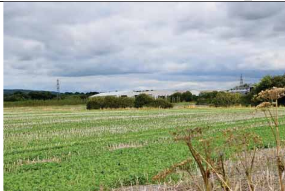
Photo 1: View from Priors Leaze Lane looking north to large farm buildings at Priors Leaze Farm
