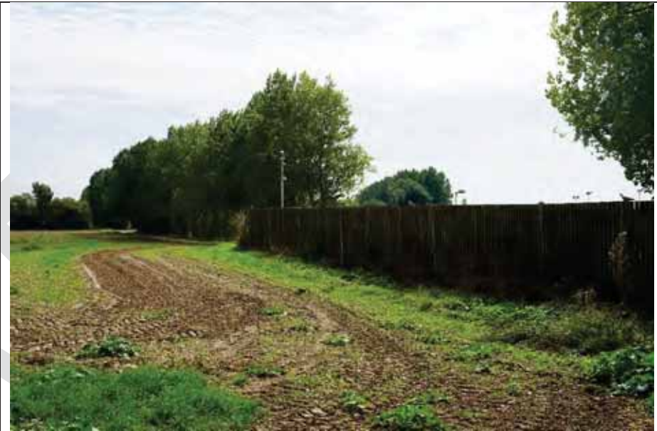
Photo 8: Boundary treatment of industrial area demarcated by close boarded fence
