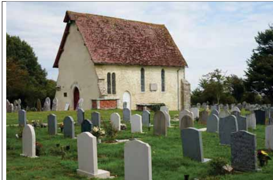
Photo 5: View of the Grade I Listed church
