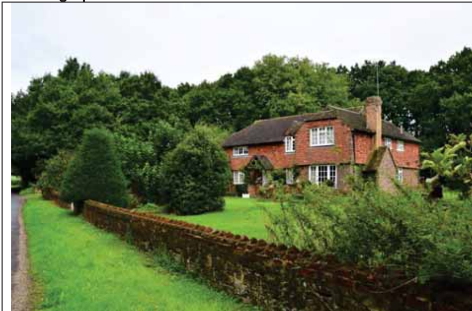
Photo 1: View north-west along Kirdford Road. Example of distinctive materials that characterise the settlement edge with wooded cover the dominant feature.
