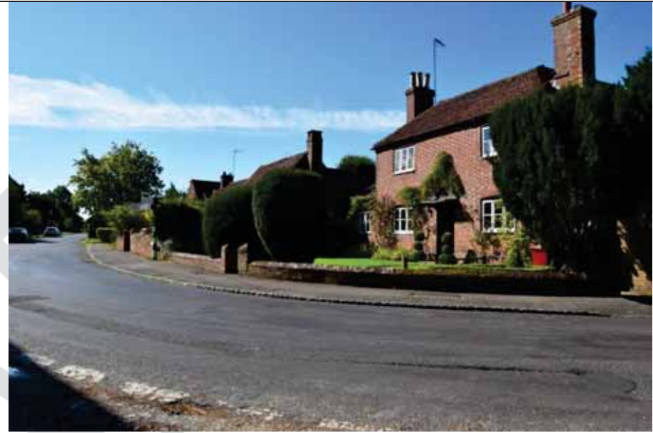
Photo 2: Characteristic buildings and boundary walls within Plaistow Conservation Area.
