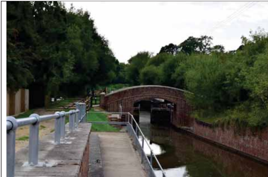
Photo 3: View west along Wey & Arun canal. Glimpsed view of landmark church with trees and vegetation along the valley floor limiting views across sub-area.
