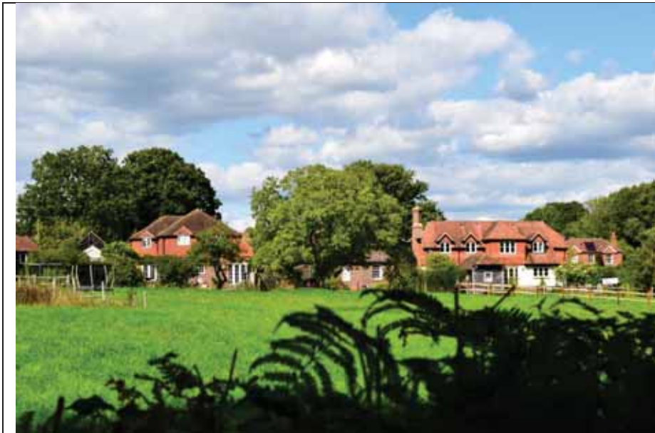
Photo 7: Modern housing set within large gardens along the southern edge of Plaistow Conservation Area.
