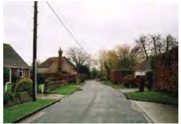
Overhead wires in Mill Lane should be removed
