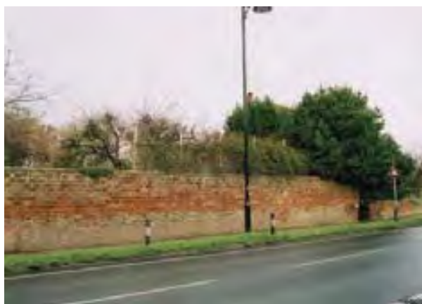
Rat trap bond brick wall in Fishbourne Road
