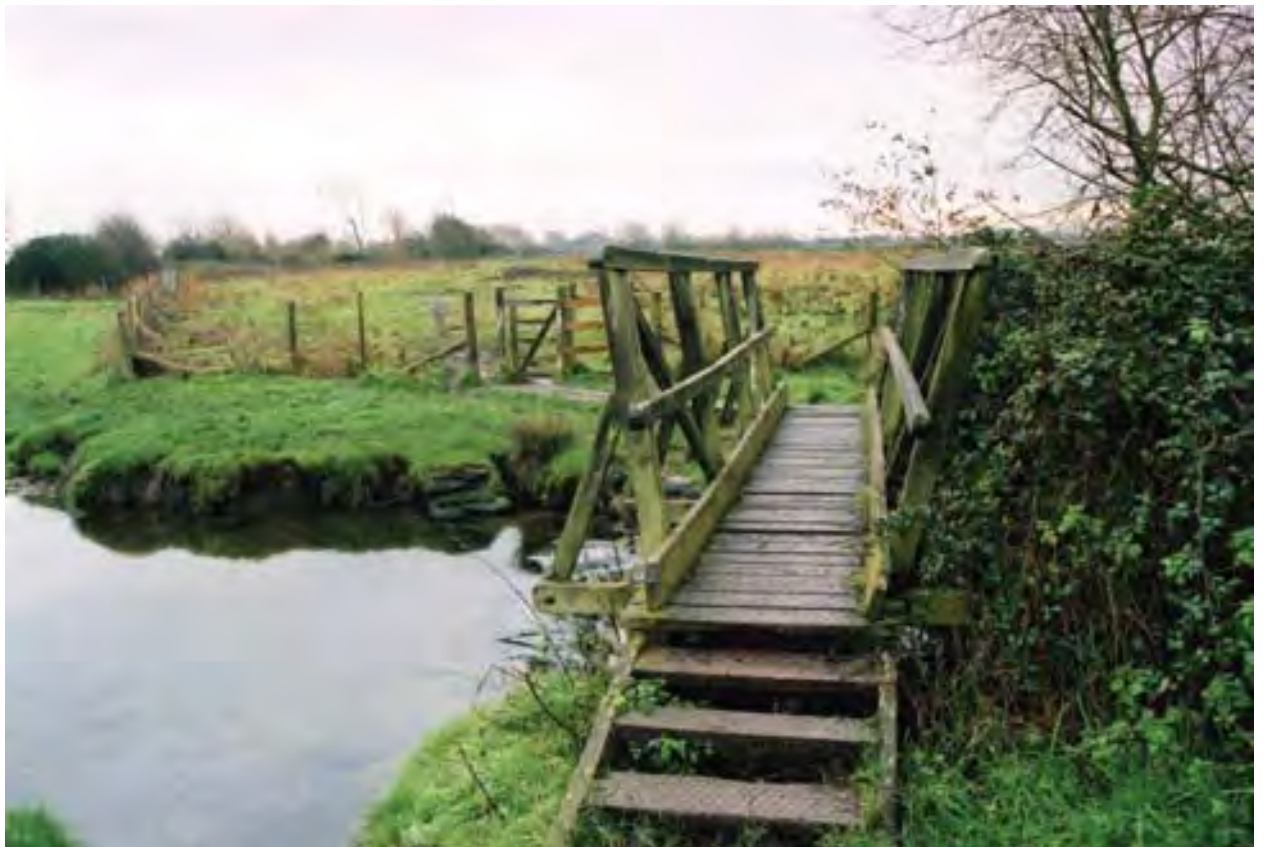
Bridge over the Fishbourne stream
