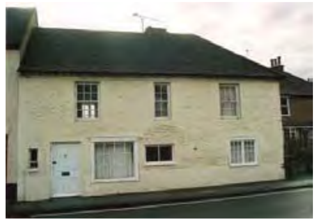
All alterations to listed buildings like this must be carefully controlled (No.87 Fishbourne Road)
