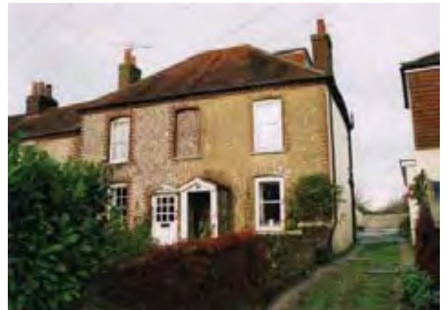
No.84 Fishbourne Road is faced in flint with red brick dressings and a handmade clay tiled roof
