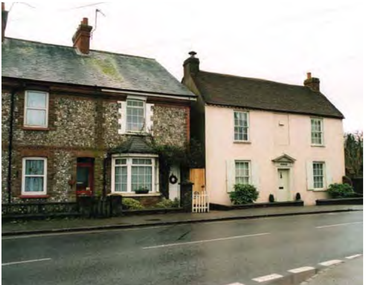
Unlisted buildings like these on the left should be encouraged to use traditional materials and details (No.111 Fishbourne Road)
