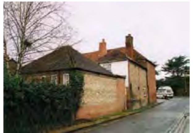
Flint and lime are important local building materials (back of the Bull's Head Public House)
