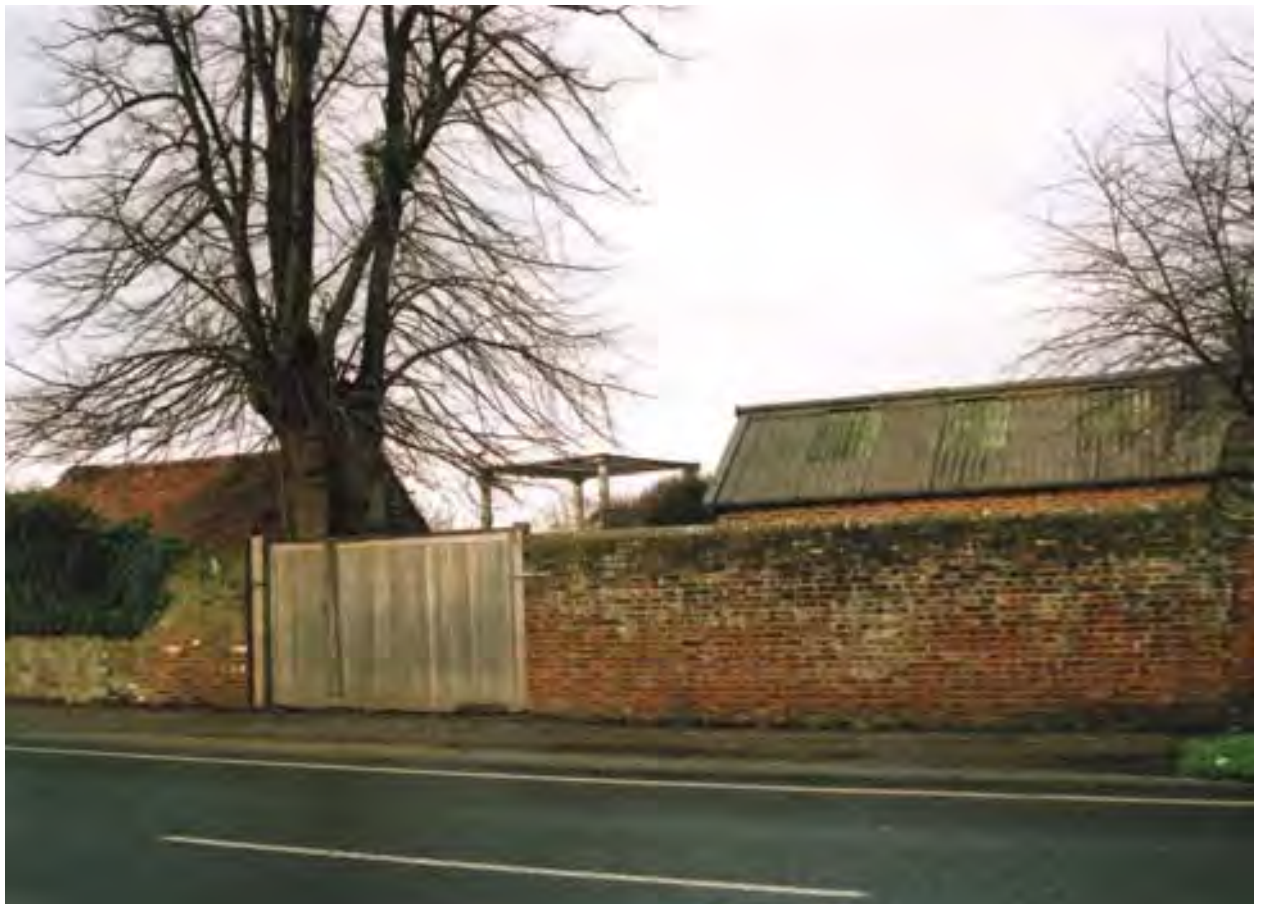
The remains of Fishbourne Palace lie to the north of Fishbourne Road
