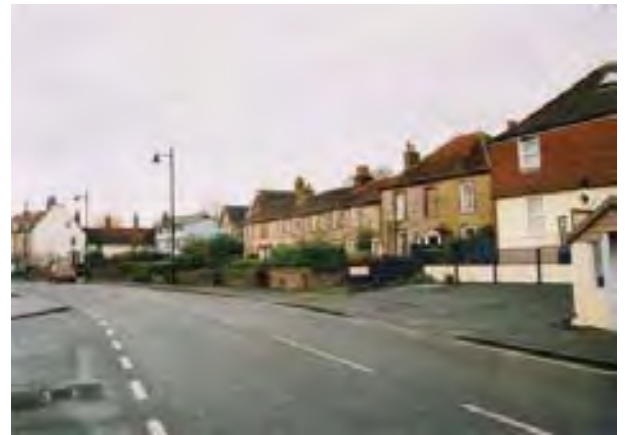
The loss of front boundaries to create parking is regrettable (No.82 Fishbourne Road)
