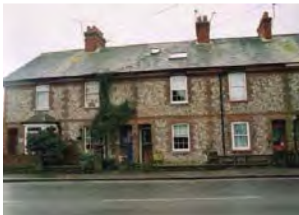
Wall outside Nos. 101 - 111 (odd) Fishbourne Road
