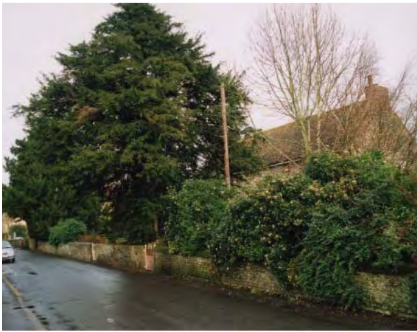
Flint walls are important (Prinsted Lane east)
