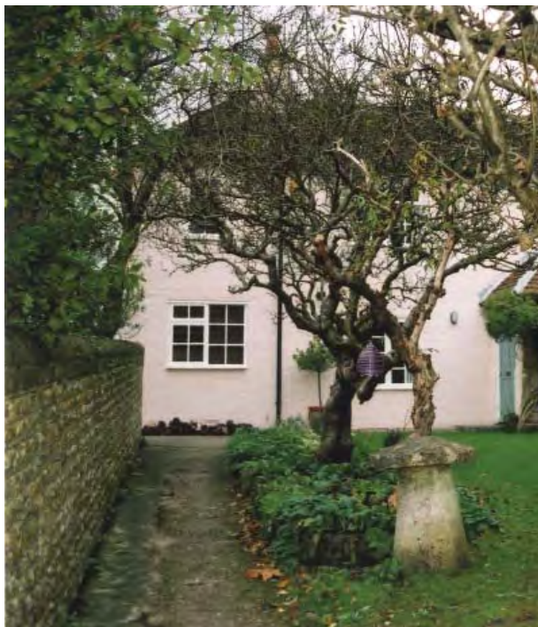
Upvc windows at Walnut Tree Cottage
