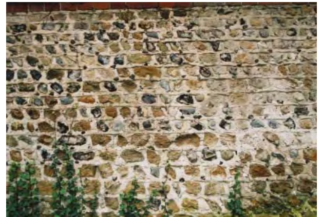
Flint walling at Pond Place, Saltham Lane
