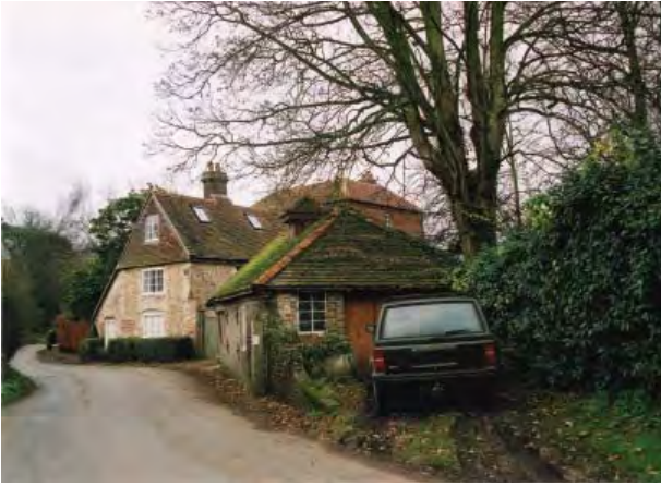
Runcton Mill, Mill Lane
