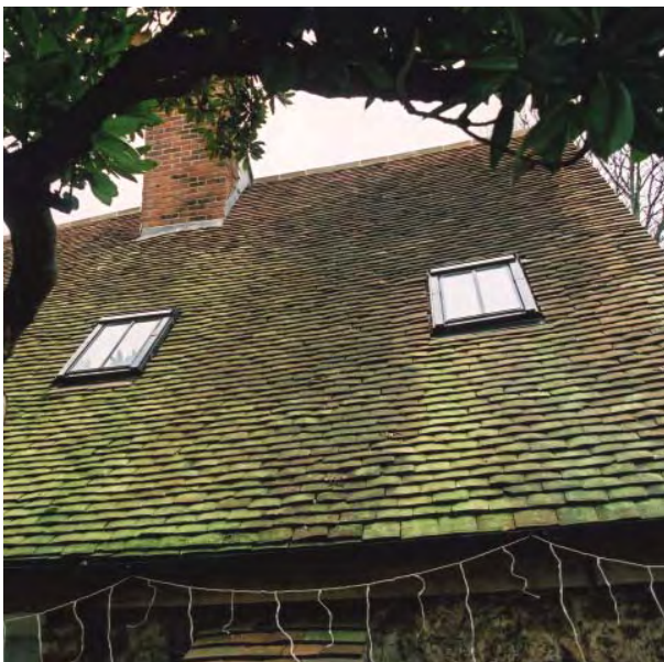
Clay roof tiles on Runcton Mill
