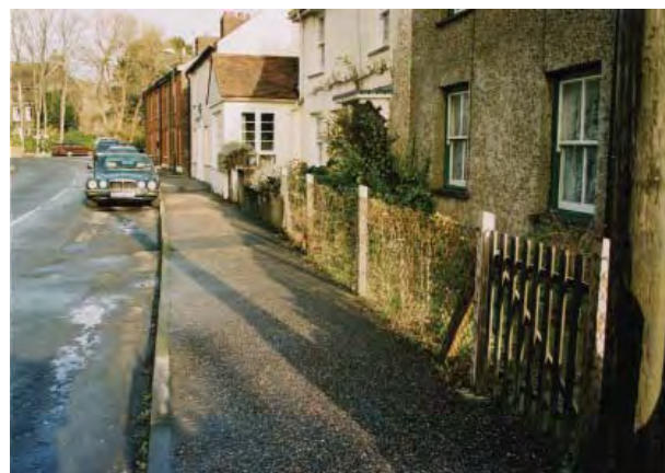
Poor quality front fence in North Street
