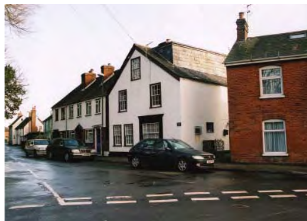
Over-sized “dormer” at No. 1a River Street
