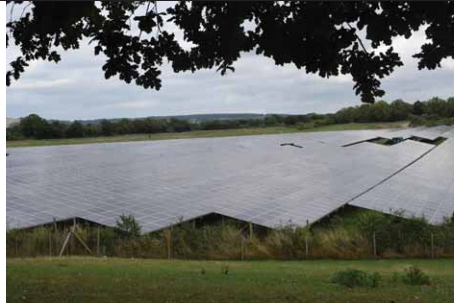
Photo 2: View across solar farm from lane north of Hunters Race within sub-area with hills on skyline within the SDNP
