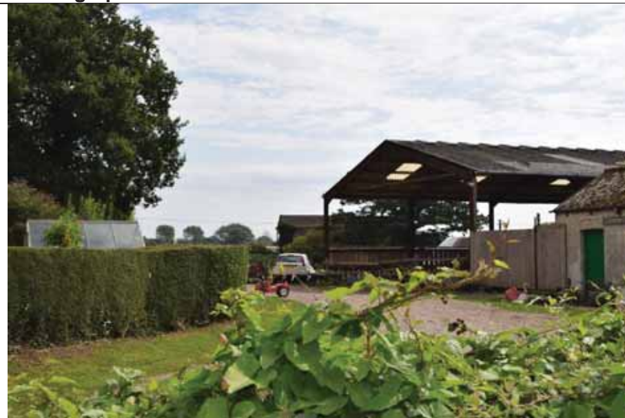
Photo 1: View east from Appledram Lane South/Salterns Way towards Manor Farm with partial views of wider landscape beyond.
