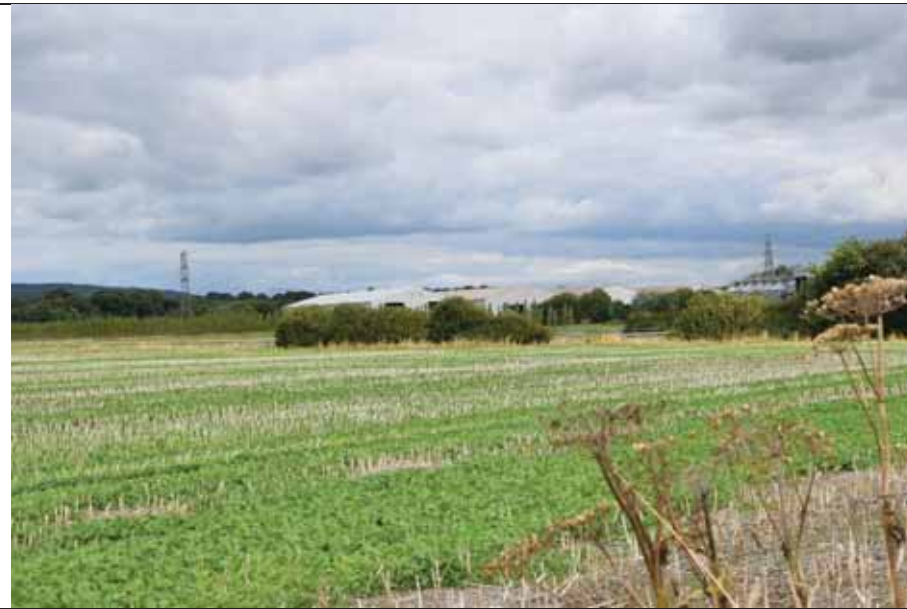
Photo 1: View from Priors Leaze Lane looking north to large farm buildings at Priors Leaze Farm
