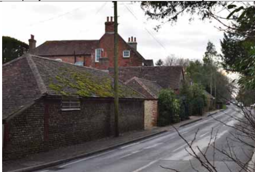
Photo 2: View south-west from B2144 Shopwhyke Road in Shopwhyke
