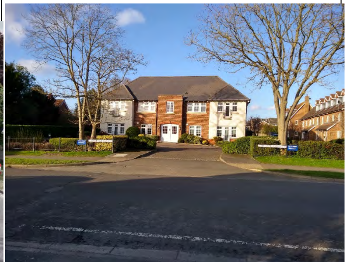
Typical junction splay for a private residential access - much too large for this location
