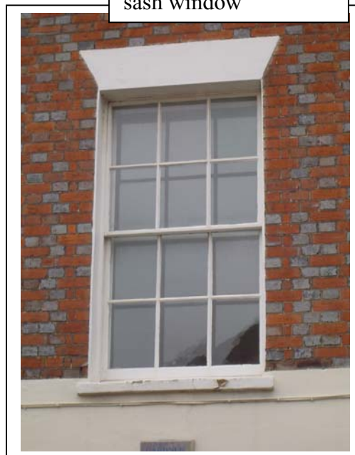
A traditional timber sash window
