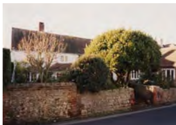
Limestone blocks form the front wall to Woodbine Cottage in Cakeham Road
