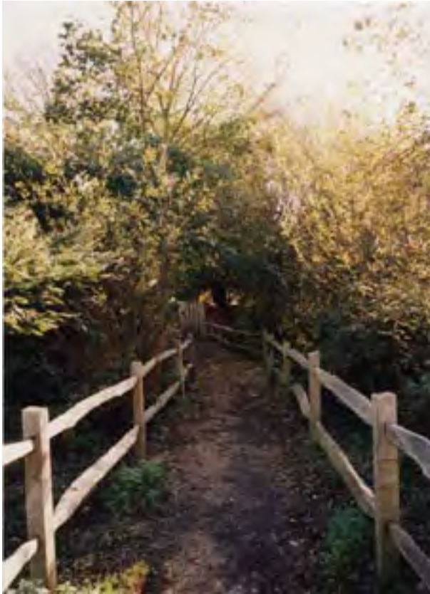
Traditional post-and-rail timber fencing to public footpath
