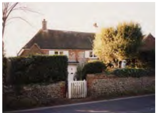
Flint is used at Apple Tree Cottage, Cakeham Road
