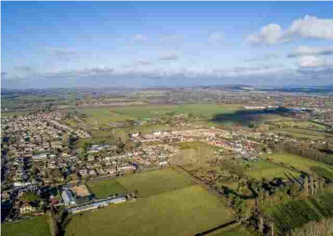
Southbourne & Land to the East - aerial picture. Credit: Angus Peel, ProAction.
