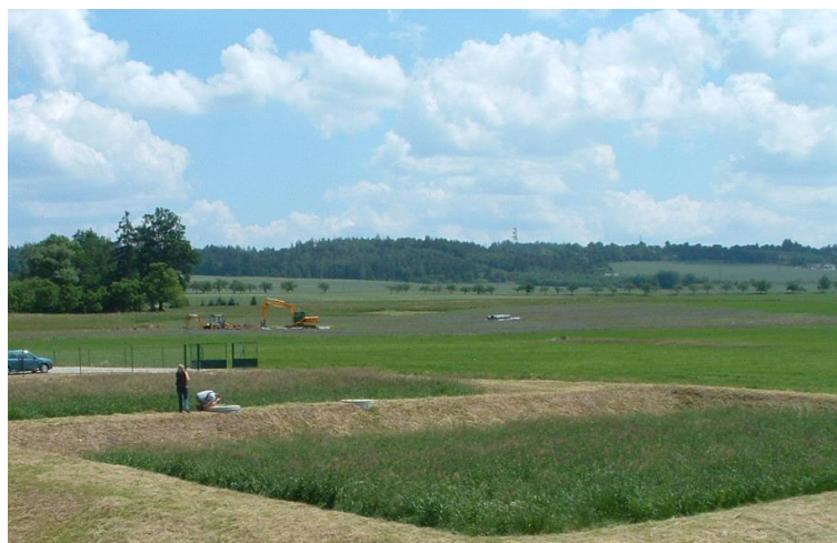
Figure 1.2 Surface flow Treatment Wetland , Czech Republic. ©R. J. McInnes
