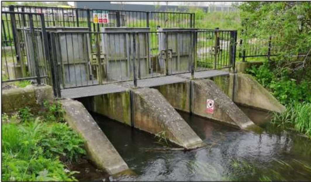
Figure 2-2: Westhampnett Mill Bypass Control Structure
