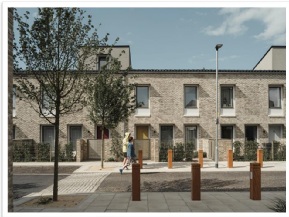
12 Passivhaus Scheme, Goldsmith Street, Norwich (Credit: Mikhail Riches)
