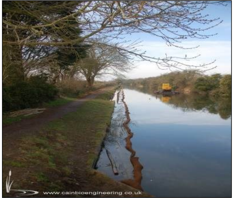
Coir fibre rolls and hazel faggots can be used to help re-narrow streams to increase water flows and restore bankside habitat
