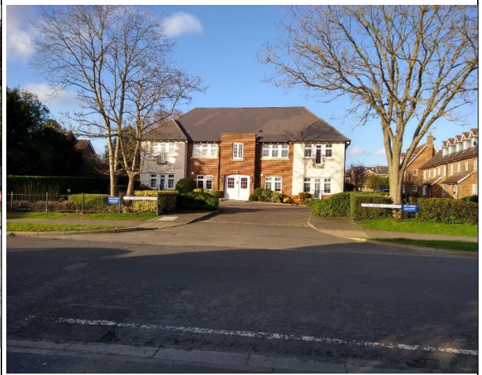
Typical junction splay for a private residential access - much too large for this location
