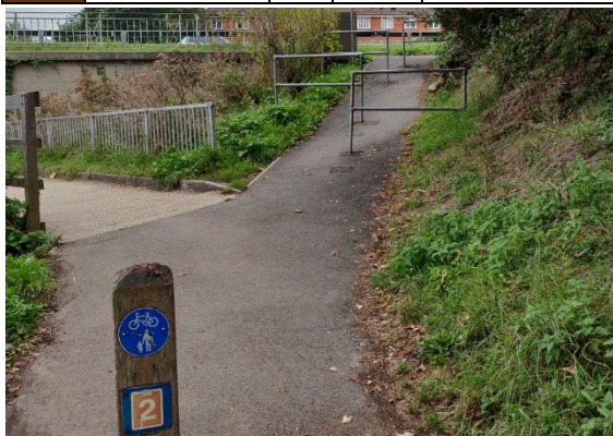
Ramp with staggered barriers between Chichester Canal towpath & A27 cycle track
