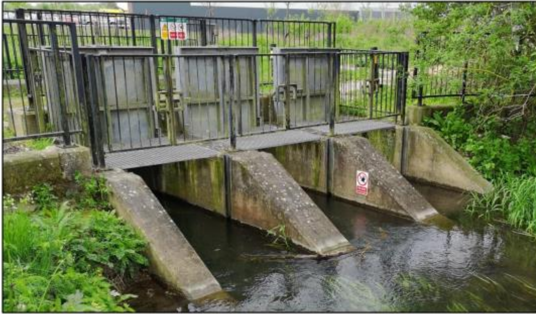
Figure 2-2: Westhampnett Mill Bypass Control Structure
