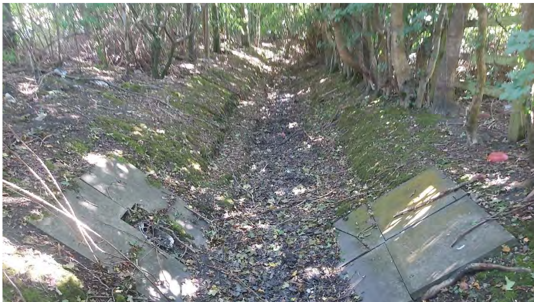
Figure 32: Existing Drainage Ditch
