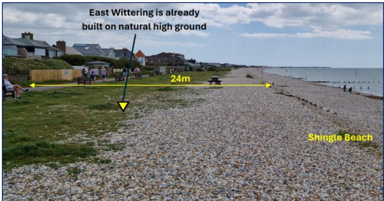
Figure 7-2: shingle beach at sea defence 75 with 74 in the background
