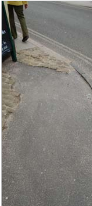
Examples of substandard footway remedial works and footways requiring maintenance
