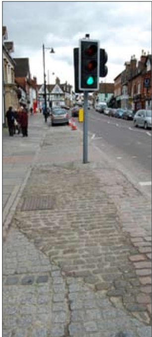
Examples of substandard footway remedial works and footways requiring maintenance
