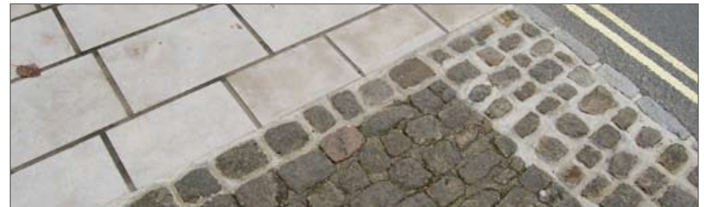
Examples of substandard footway remedial works and footway improvements
