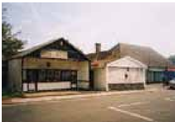
These buildings need to be sensitively redeveloped (Nos. 71 & 73 High Street)
