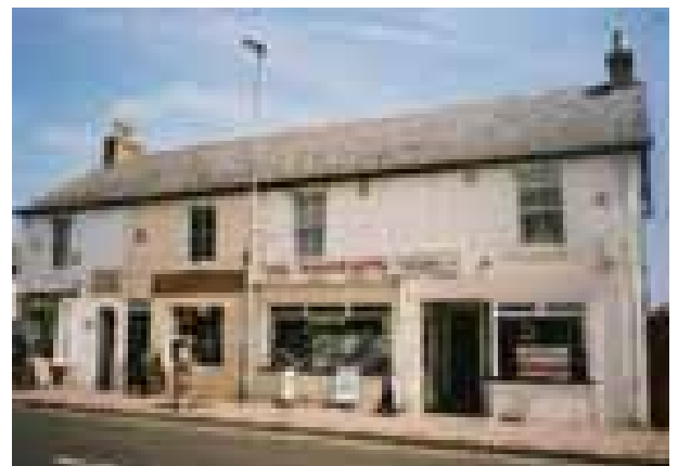
“Positive” buildings in the High Street (Nos. 68 - 72)
