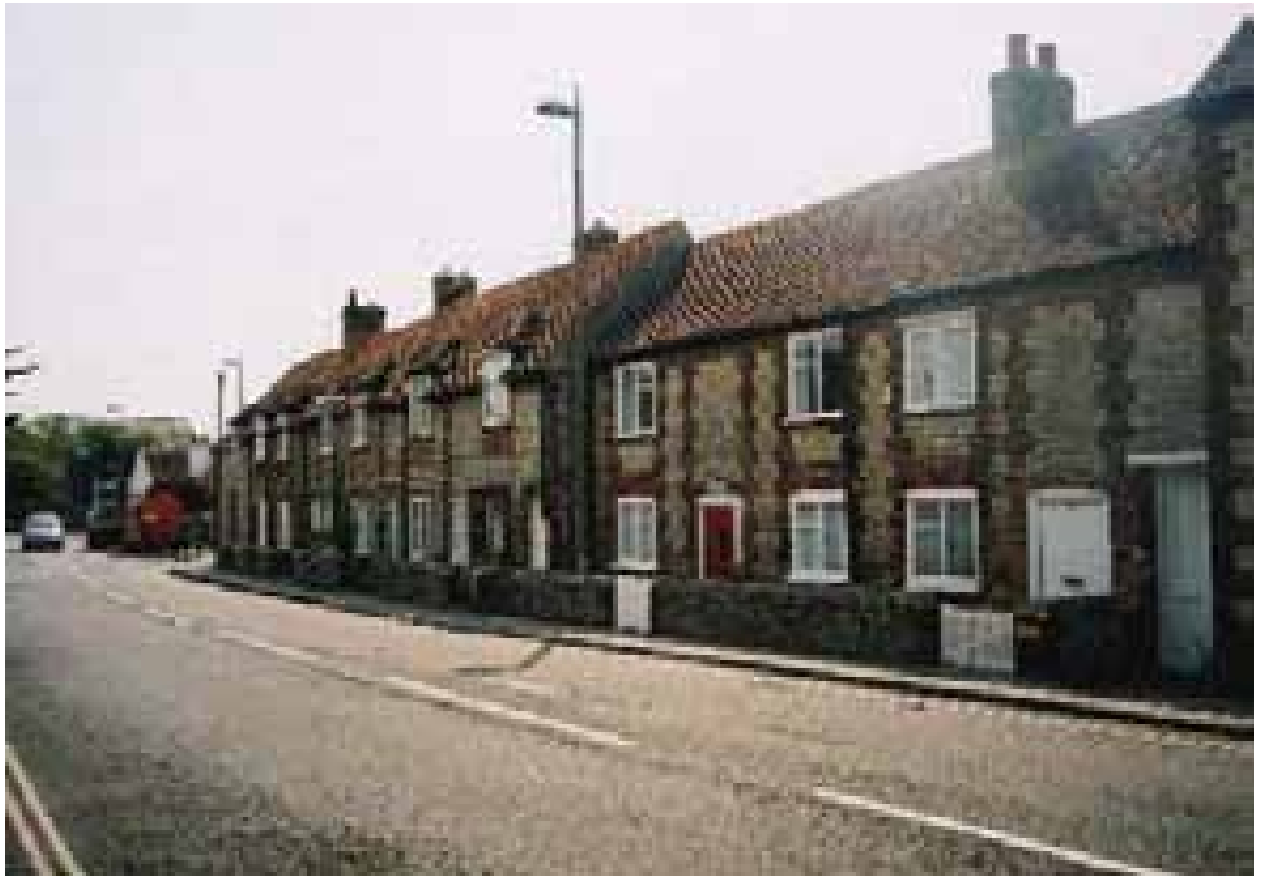
Orangey / brown clay tiled roofs are a significant feature
