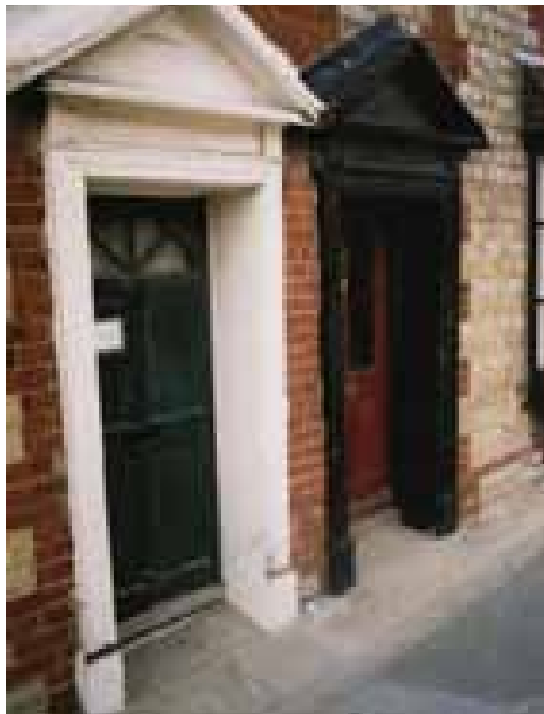
Georgian doorcases to Nos. 24 and 26 High Street
