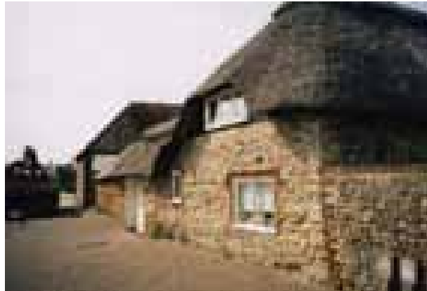
Mixer Stone, brick and beach flints are used in Hollyhocks and the adjoining listed barn
