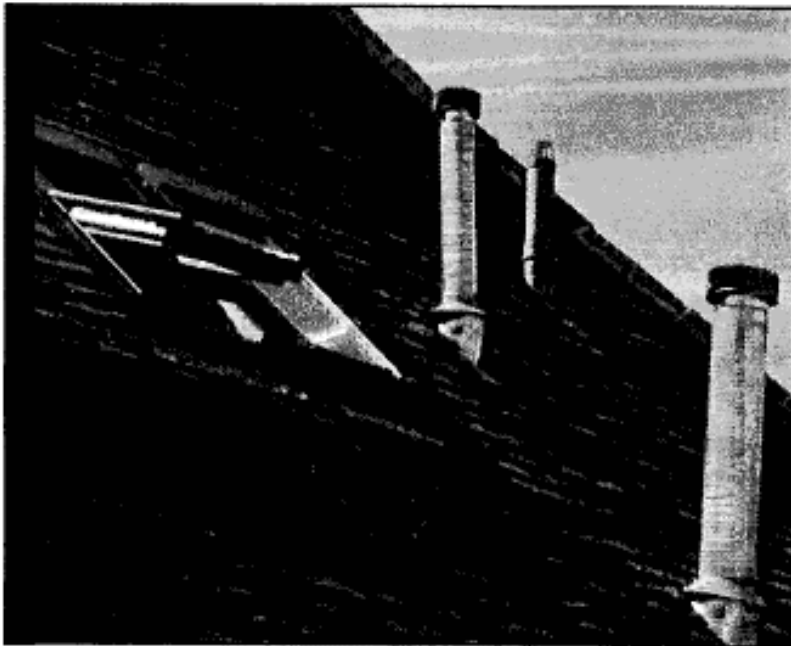
Unsightly ventilation pipes and flue pipes
