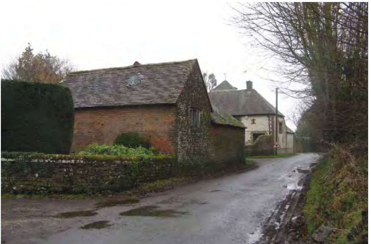
The barn next to North End Barn
