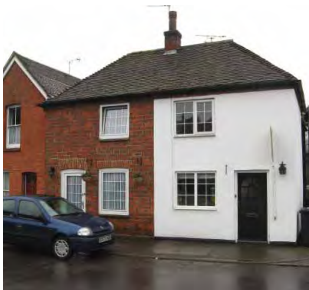
These unlisted buildings facing The Square could be protected by an Article 4 (2)
