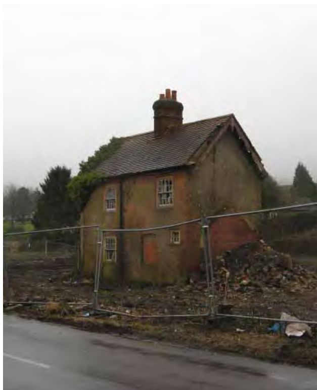
Former Smithy Site, Elsted Road
