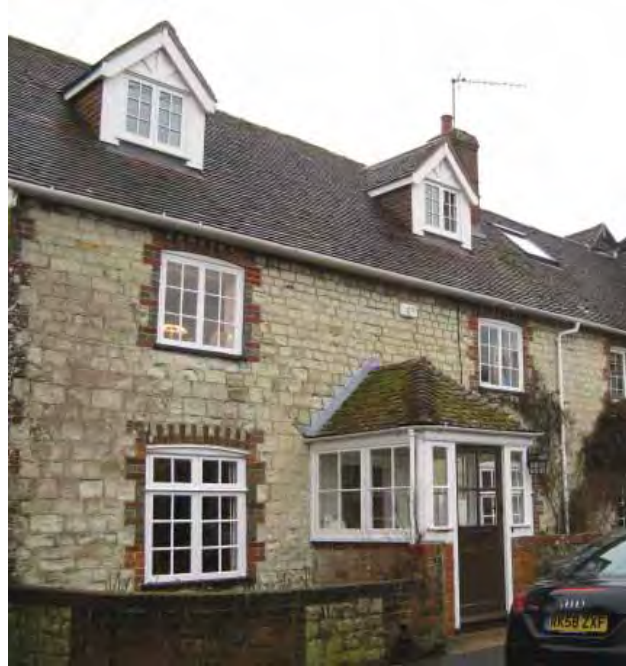
Glazed porch on North Way, North Lane
