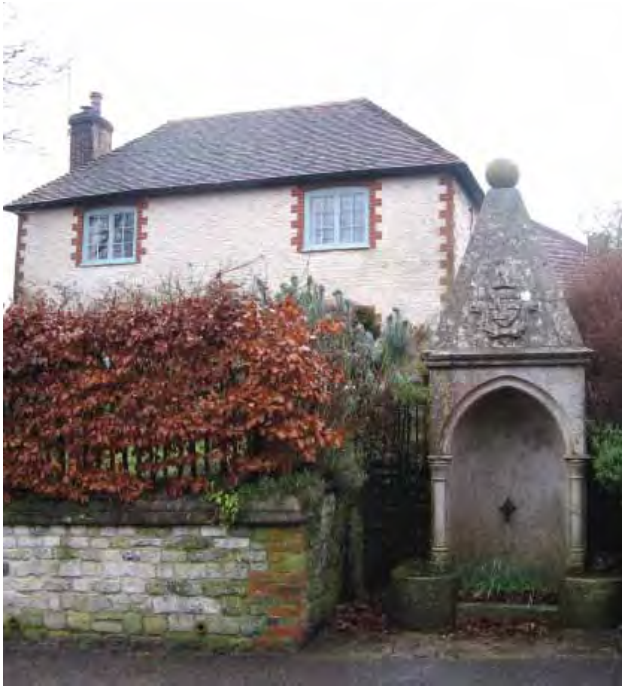
The Postlethwaite pump in North Lane
