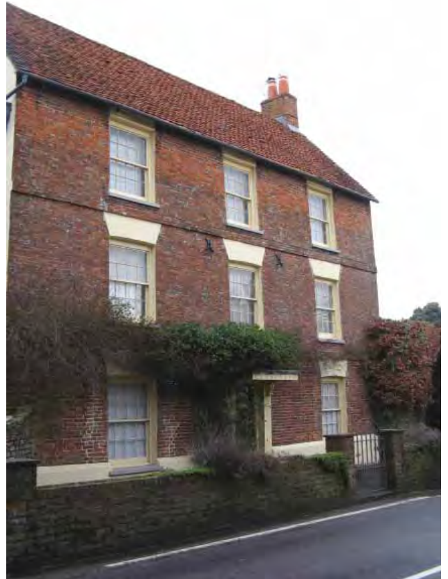
The High House, Petersfield Road
