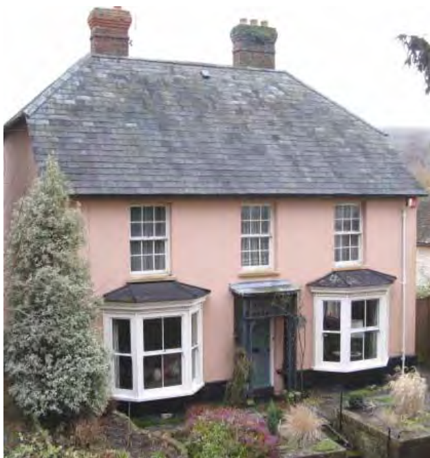
This unlisted house in The Street is unusually covered in Welsh slate
