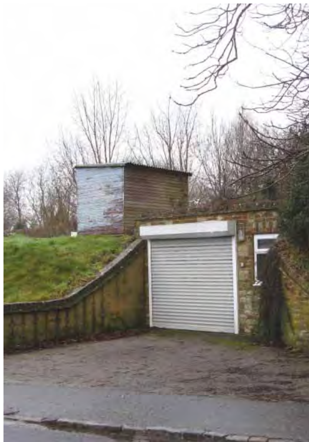
A modern garage in North Lane
