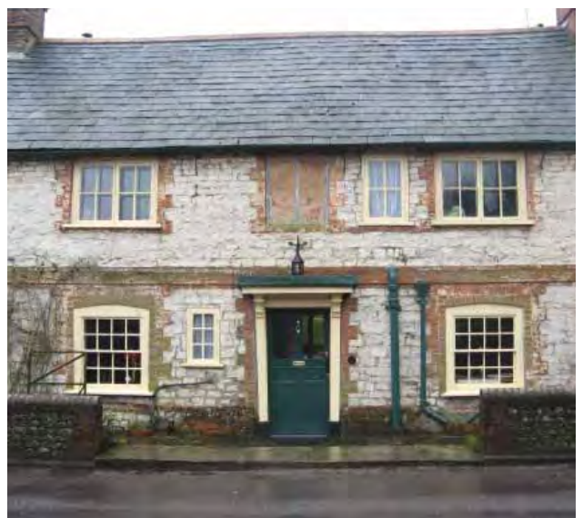
The Cottage, Elsted Road
