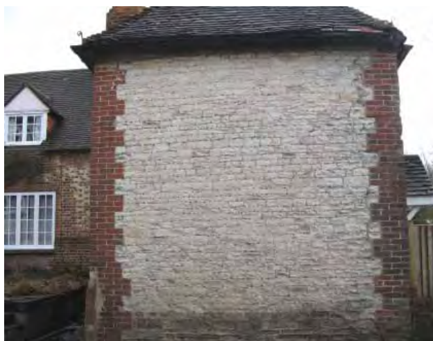
Brookside Cottages - galletting on flank wall
