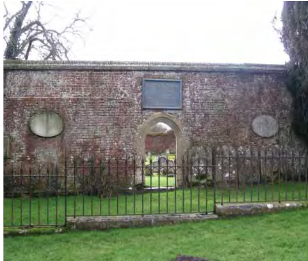
One of the brick walls around the churchyard
